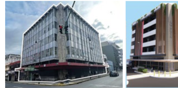
▲ Figure 10. Retrofit of Amalia building. © Jocelyn Jiménez | San José RISE project
